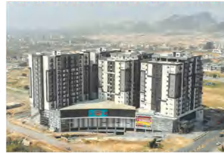
Capital Square (27 Kanal Mall & Apartments) B-17, Islamabad
